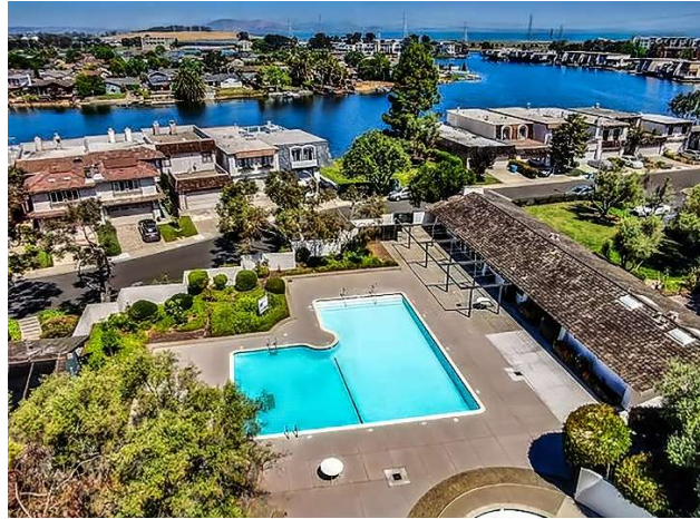
Mariners Green 2 Clubhouse Pool Complex
